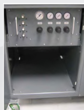
Air Adjustments & Storage Area
